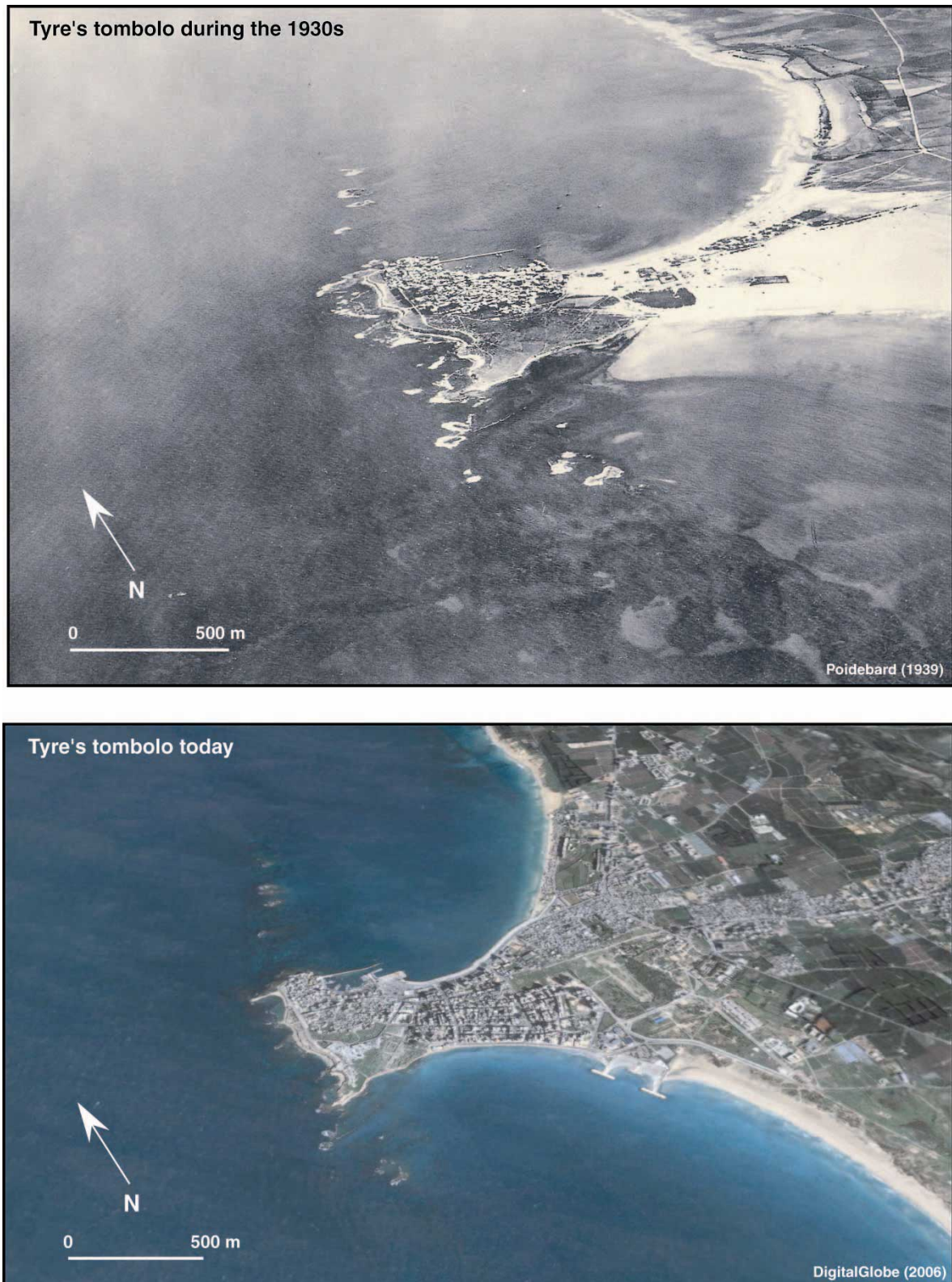
Figure 2.8: Twentieth century evolution of Tyre's tombolo. While the dimensions of the tombolo have remained relatively stable, the sandy salient has been extensively urbanised since the 1970s. This surface construction work has led to a loss of the surficial medieval and modern period geological records.
