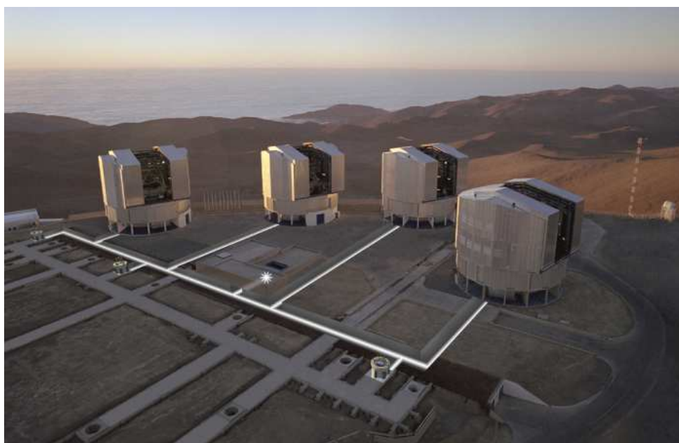
Figure 5: The ESO Very Large Telescope Interferometer with its four 8-m Unit Telescopes, three of its four 1.8-m Auxiliary Telescopes (artist impression) and its central beam combining laboratory (© 2000, ESO).
