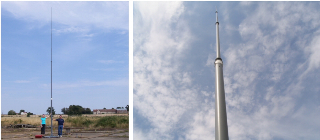
Figure 2.1: Example of HF quarter wavelength monopole antennas
